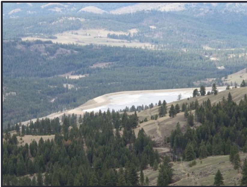
View of tailings pond from Adamera's Oversight project
